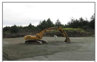
Work continues at the Millstream Meadows site in south Highlands. Pictured is the portion of the excavation that is currently being in filled. The pipe will be a recovery well, located at the deepest point, that will be used to capture any remaining hydrocarbon contaminants . A consultant's report, to be received by the CRD Environmental Sustainability Committee soon, is expected to provide recommendations for further remediation of the site.
