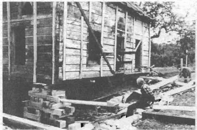
A replacement log being slid into place during restoration of the Pike House.
