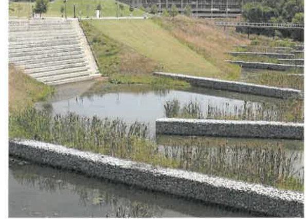
Constructed wetlands provide aesthetic and educational benefits while they utilize remove contaminants and provide wildlife habitat.
