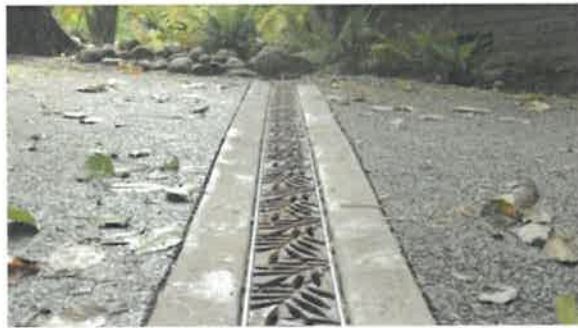
Grates allow stormwater to pass through while allowing for pedestrian movements.
