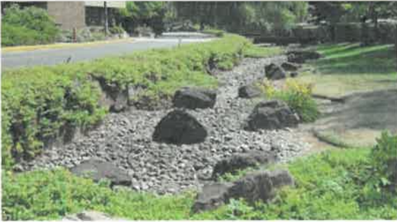
Rain gardens have been shown to decrease the temperature of runoff from certain land uses, such as parking lots and roadways.
