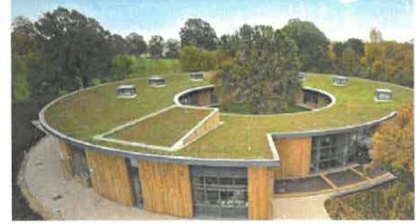
Green roofs store and utilize stormwater to reduce runoff from building sites.
