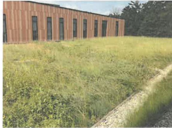
Green roofs provide shade, remove heat from the air, and reduce temperatures of the roof surface and surrounding air.
