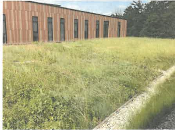
Green roofs provide shade, remove heat from the air, and reduce temperatures of the roof surface and surrounding air.
