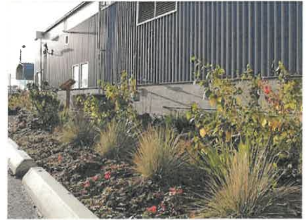
Bioswales reduce stormwater run-off.
