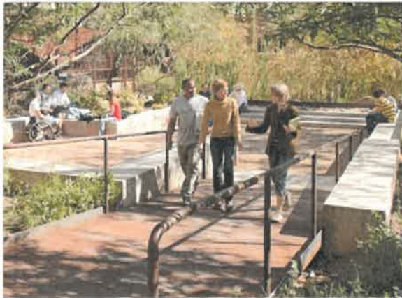
Outdoor space with garden/outdoor classroom provide cleansing gardens for adjacent buildings and pavement runoff.
