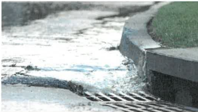
Example of an EIA - precipitation falling and flowing to a stream along a continuous impervious pathway.
