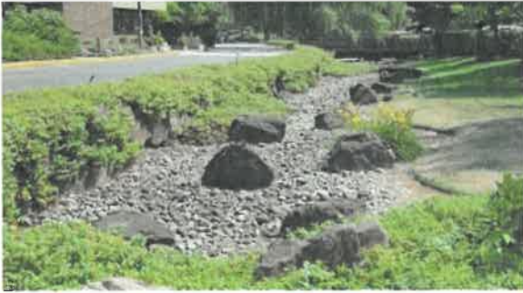
Rain gardens have been shown to decrease the temperature of runoff from certain land uses, such as parking lots and roadways.
