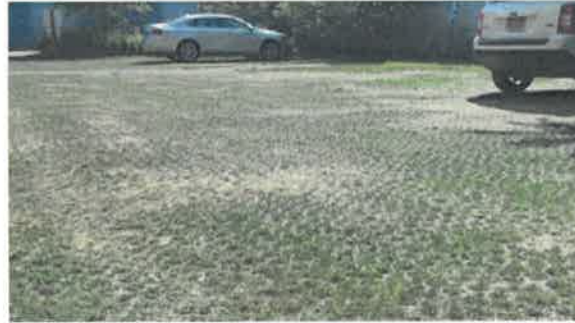
Structural grid paving reduces runoff in parking areas.
