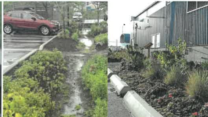
Example of a non-EIA - precipitation flowing into an area of a parking lot that mimics natural hydrology.
