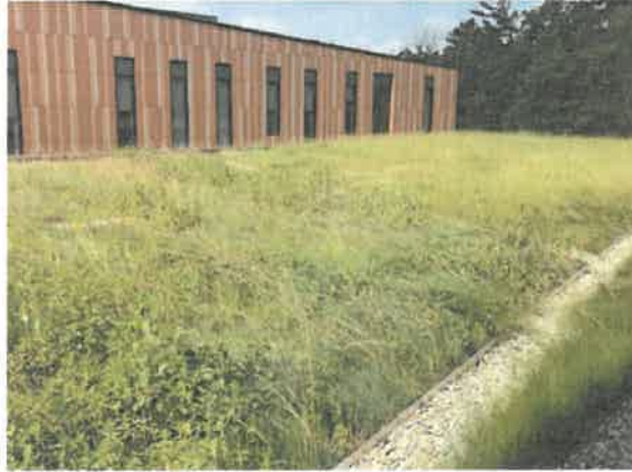
Green roofs provide shade, remove heat from the air, and reduce temperatures of the roof surface and surrounding air.
