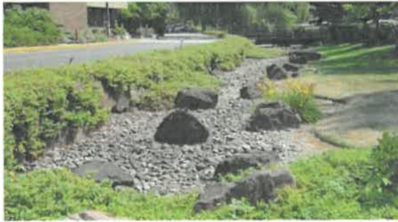
Rain gardens have been shown to decrease the temperature of runoff from certain land uses, such as parking lots and roadways.
