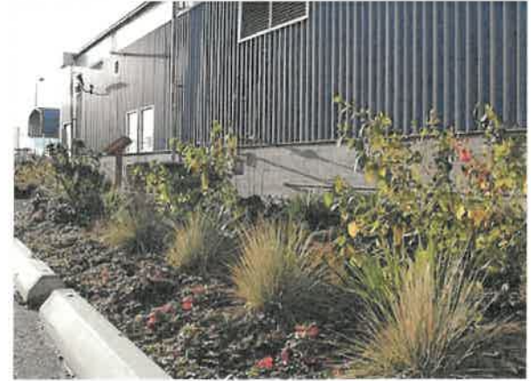
Bioswales reduce stormwater run-off.
