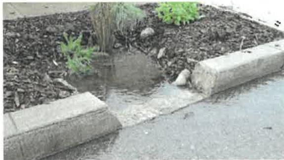
Curb cuts direct stormwater from street to landscape areas.
