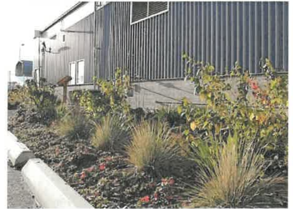
Bioswales reduce stormwater run-off.
