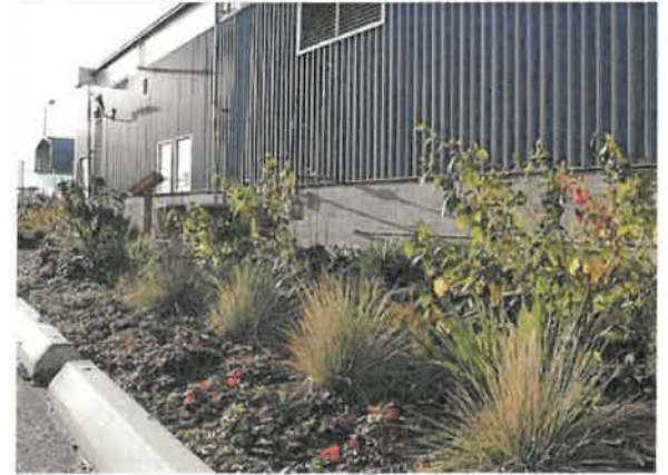
Bioswales reduce stormwater run-off.
