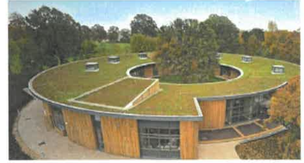
Green roofs store and utilize stormwater to reduce runoff from building sites.
