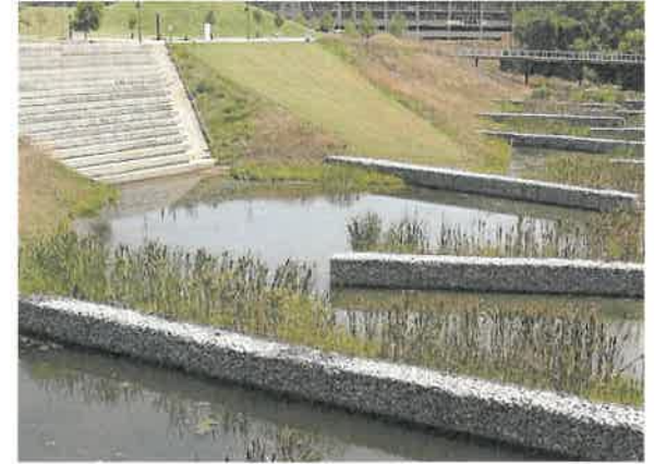
Constructed wetlands provide aesthetic and educational benefits while they utilize remove contaminants and provide wildlife habitat.
